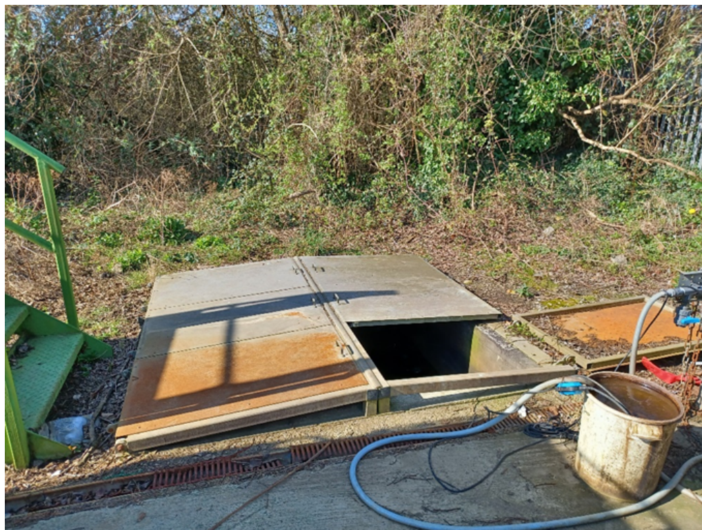
Image 3: Surface water sump associated with the drainage infrastructure of the Rear Compound.
