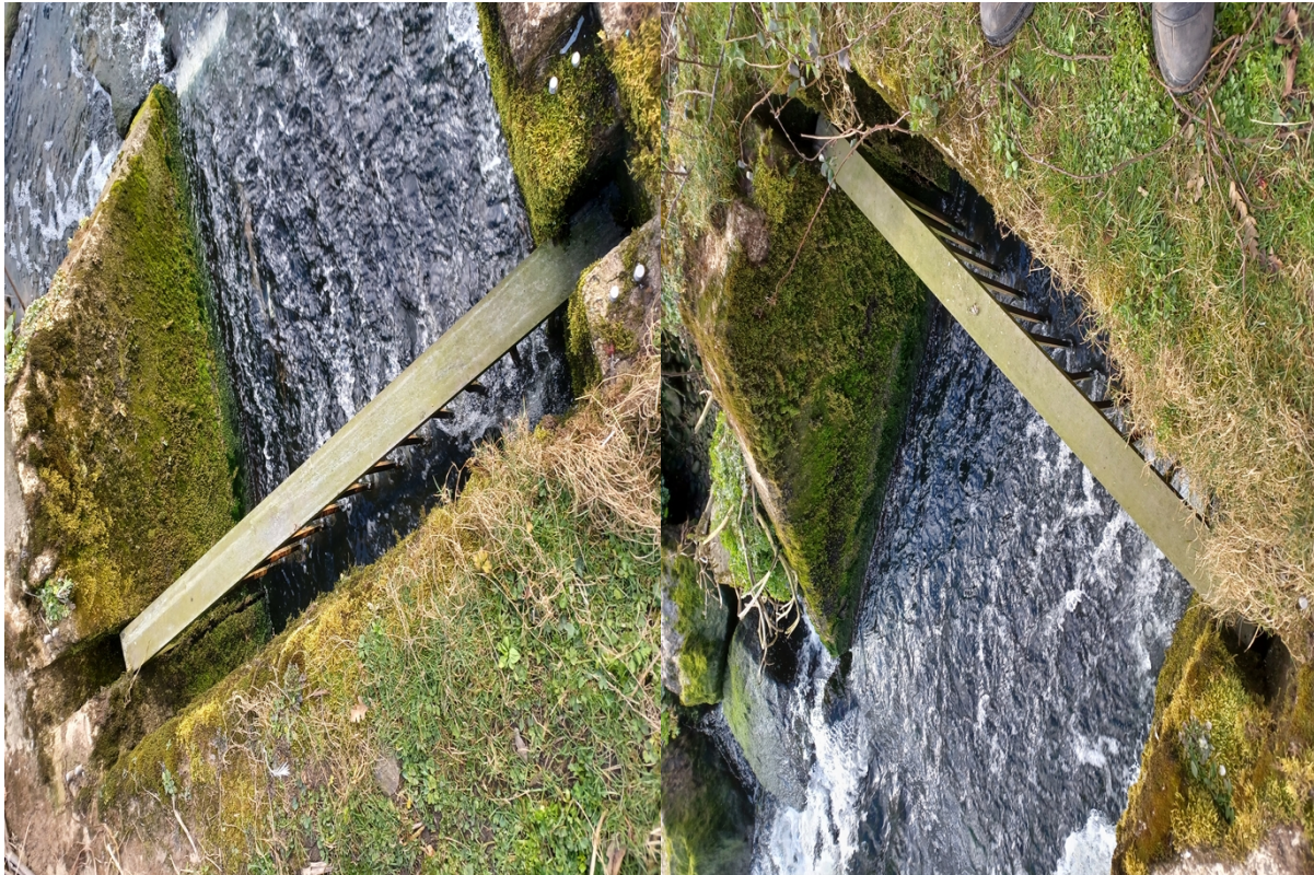
Figure 1 and 2 - screens at discharge point
