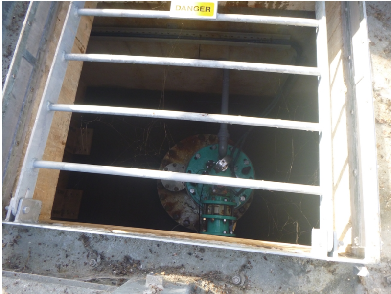
Figure 1: Point A underground chamber
