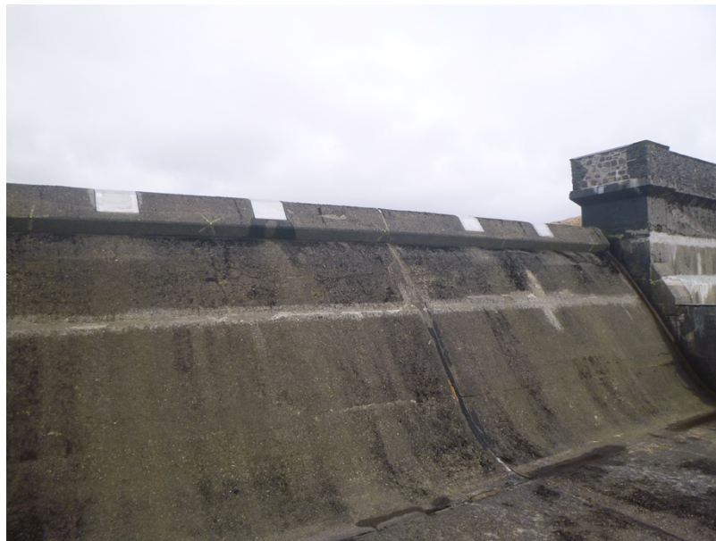
Figure 1: Llyn Egnant dam wall
