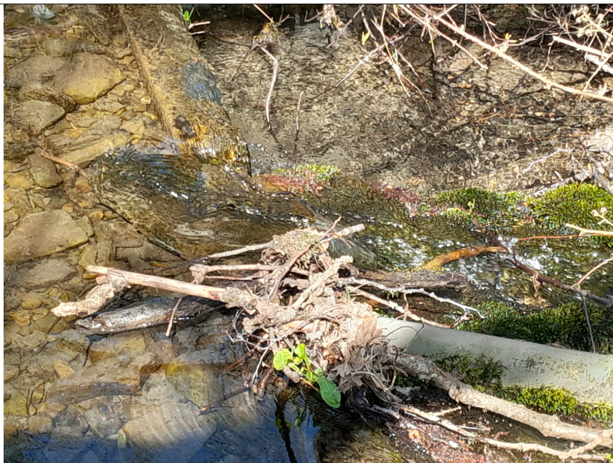
Image 2: Compensatory flow notch and fish easement.
