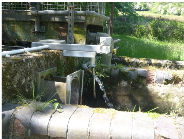
Photograph 1: New EDM radar unit on site
