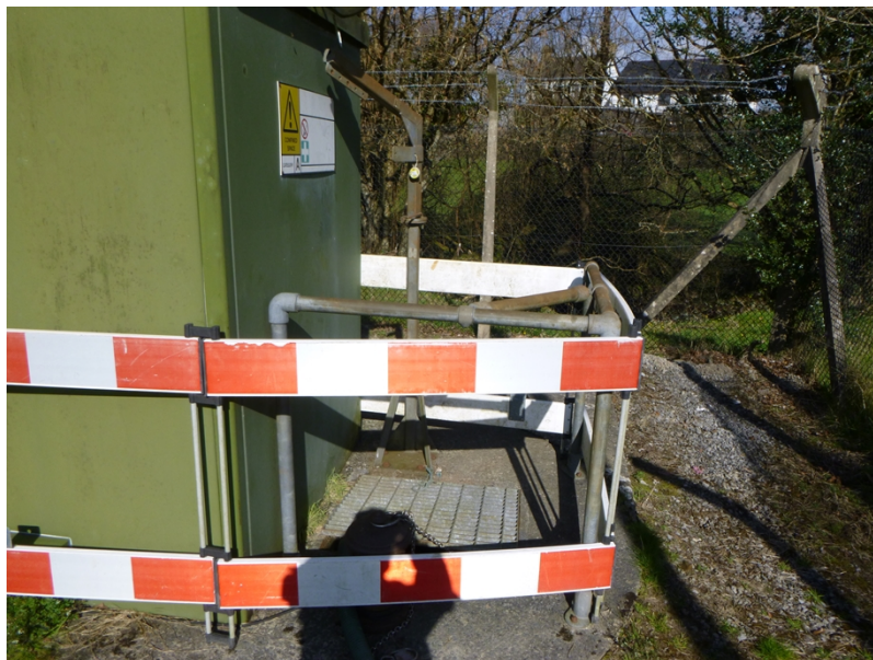
Photograph 1: Rhydlewis PS No 1. Wet well exists below grate.
