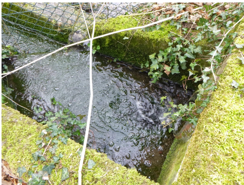
Photograph 11: Final effluent and storm discharge outfall into the Nant Medini
