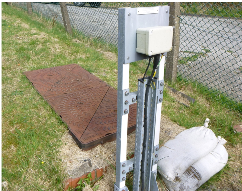
Photograph 2: EDM monitor
