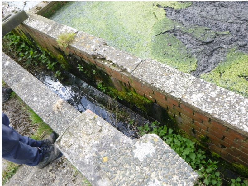
Photograph 7: Effluent channel beside sludge holding tank
