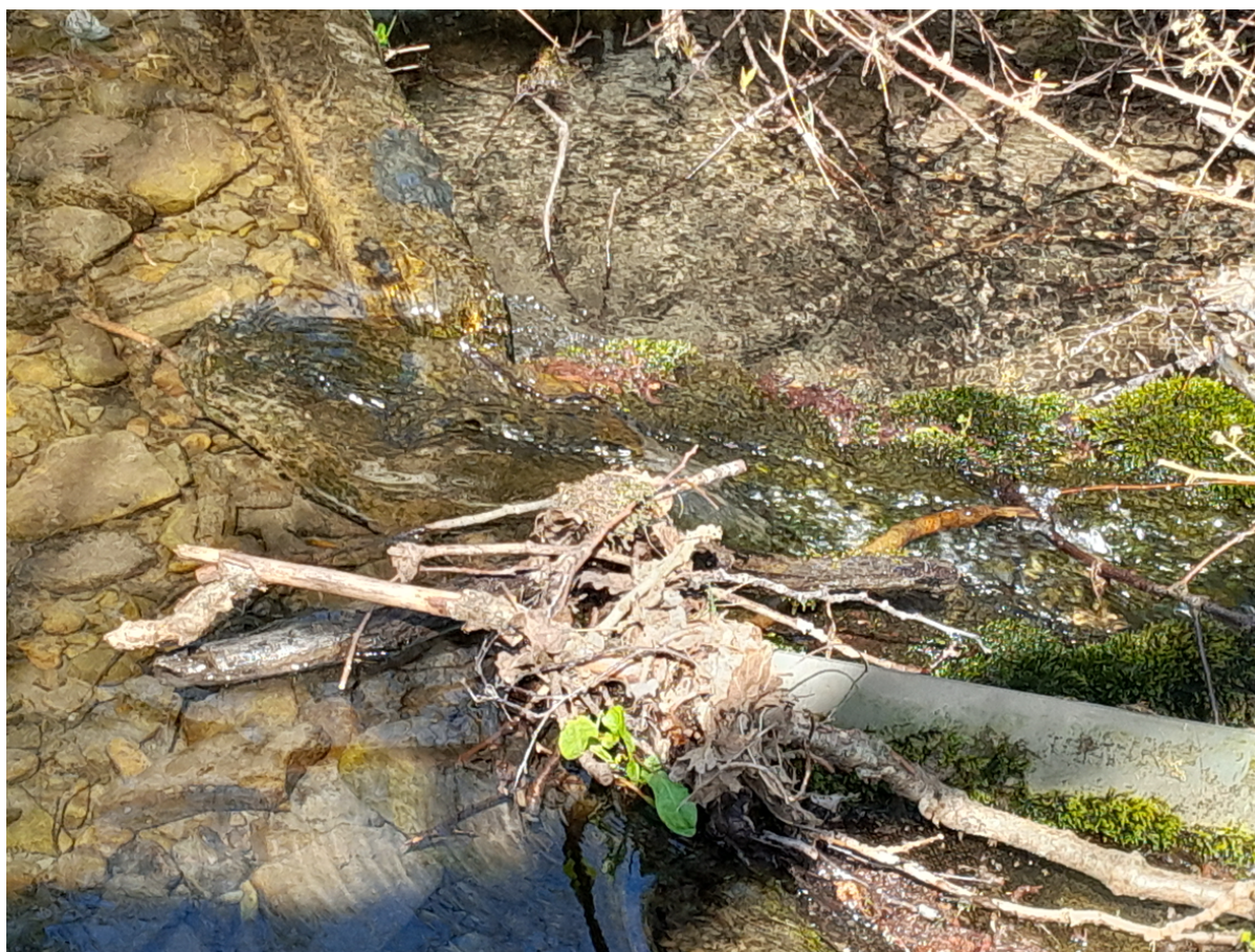
Image 1: Compensatory flow notch and fish easement.
