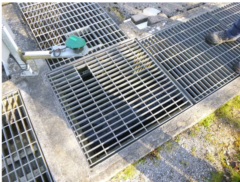
Photograph 1: Rhydlewis WwTW inlet and EDMS monitor
