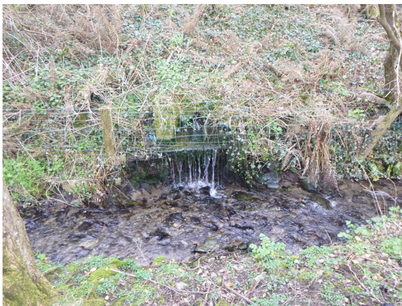
Photograph 10: Ferwig STW's final effluent and storm outfall into the Nant Ferwig
