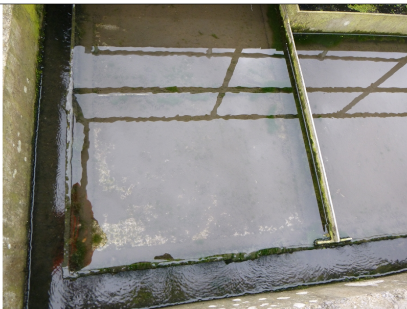
Photograph 6: Second settlement tank
