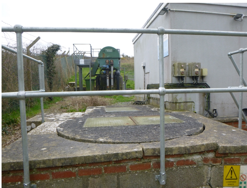
Photograph 1: Inlet chamber at Ferwig WwTW
