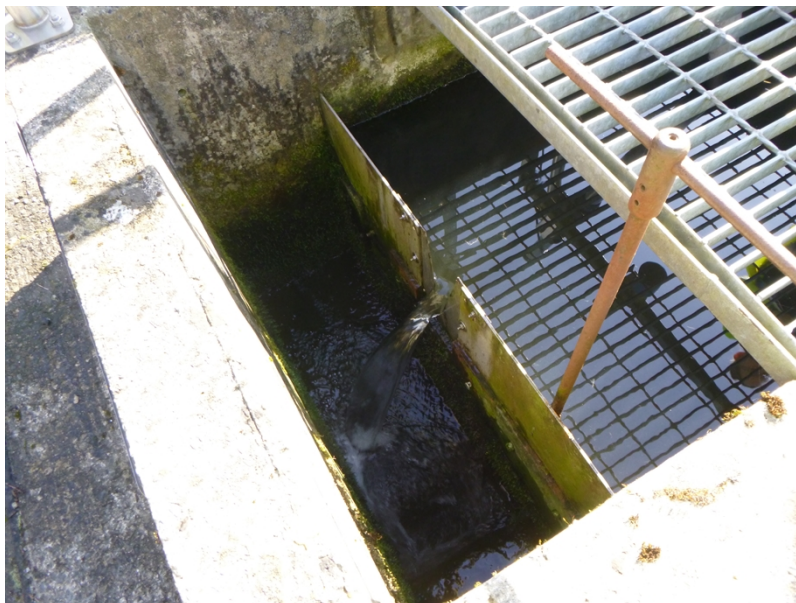
Photograph 4: Final effluent at Rhydlewis WwTW
