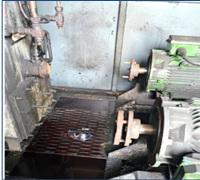
Photo: hydraulic pump removed from battery machine
