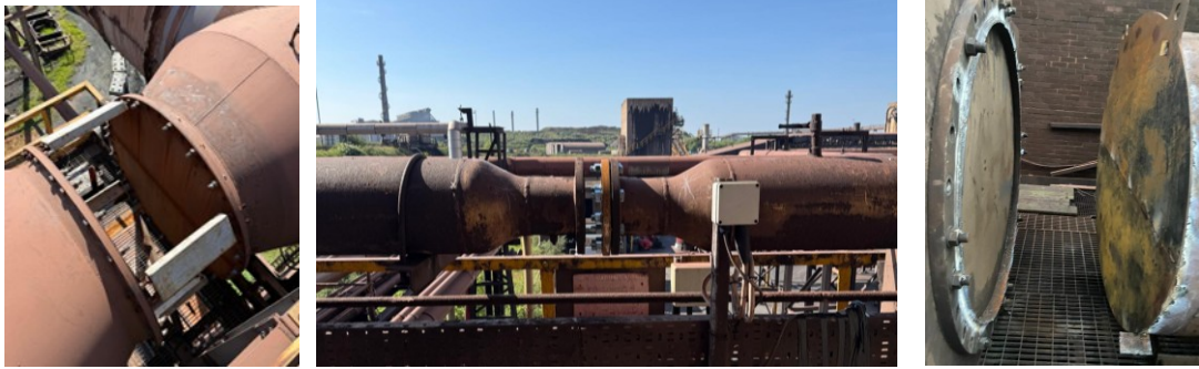
Photo : process gas pipelines cut and blanked with line of sight
