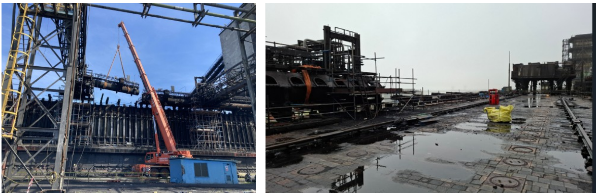
Photo: removal of unstable gas pipes from the battery top
