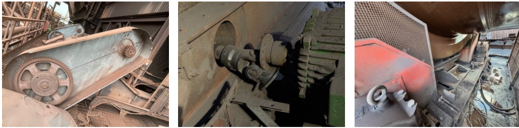
Photo: drive chain removed, screen drives disconnected, mixer immobilized
