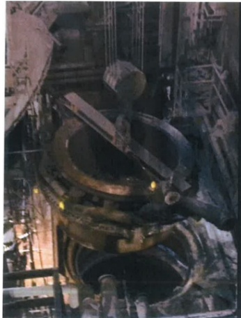
Photo: lower hood being removed from vessel
