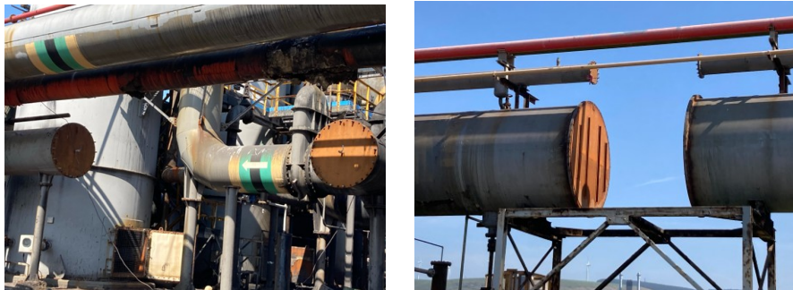
Photo: section of process gas transport removed
