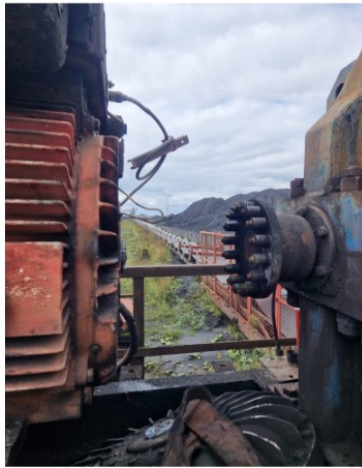
Photo: Conveyor 804, coupling in drive removed and Conveyor 801 electrical supply cut and capped
