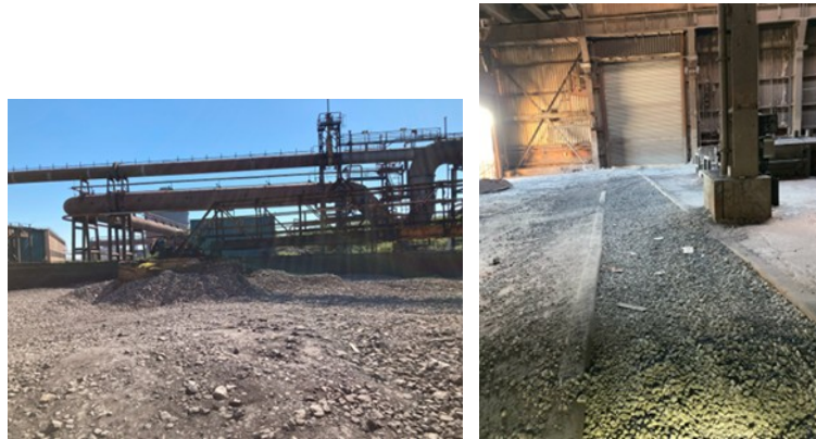
Photo : water separation pond and slag runner filled up with stone
