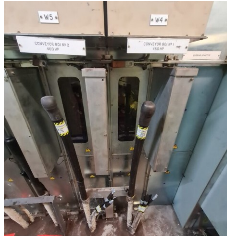
Photo: Conveyor 804, coupling in drive removed and Conveyor 801 electrical supply cut and capped
