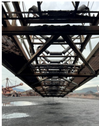
Photos: Conveyor Belt removed from Ore Stacker
