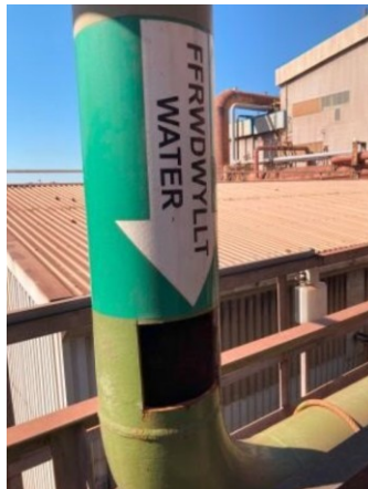
Photo : Water supply pipe cut to Demineralisation Plant decommissioned
