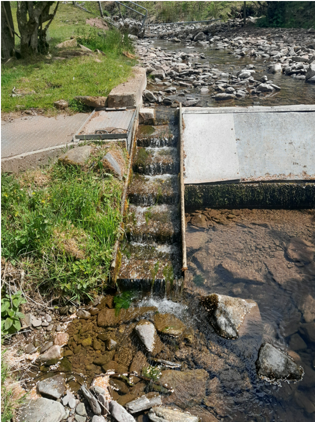
Photograph 1: Please remove material from below the fish pass to create a plunge pool to aid fish passage.
