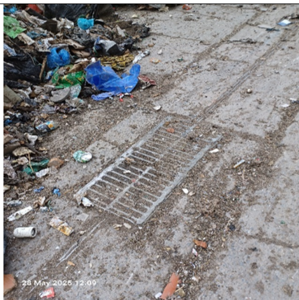
WTS Linear drain
