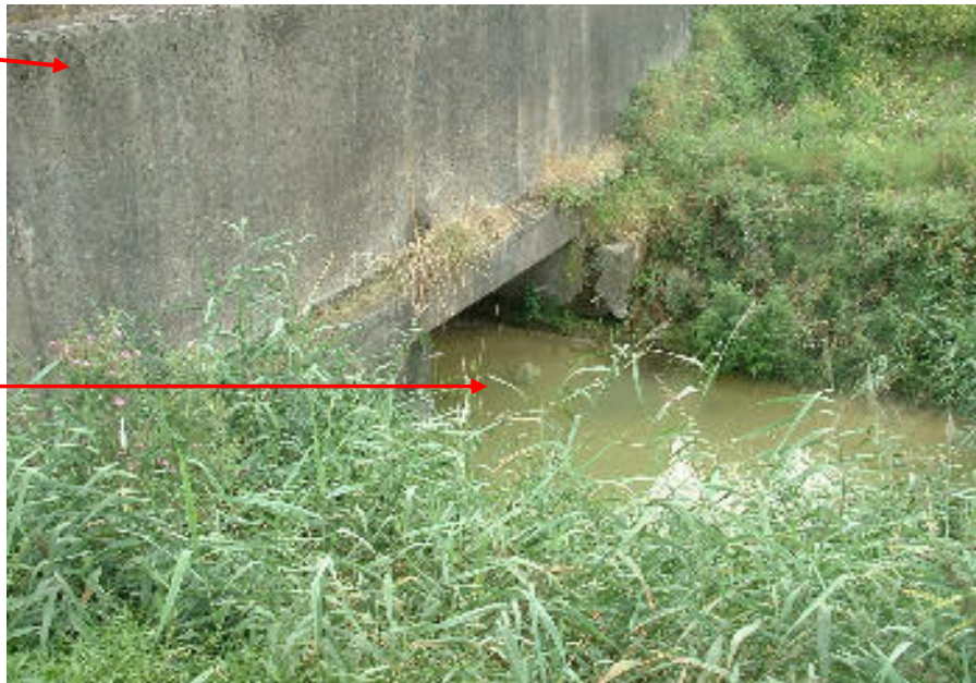
Photo 5: Main east west ditch culverted under Monks Ditch.
