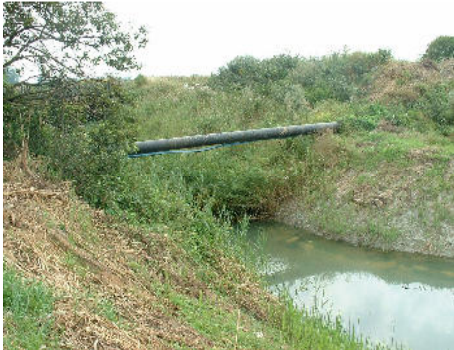
Photo 3: Service pipe crossing main East-West Ditch at the southern end of the site.
