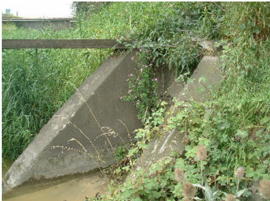
Photo 2: Drain outfall into main East-West ditch.
