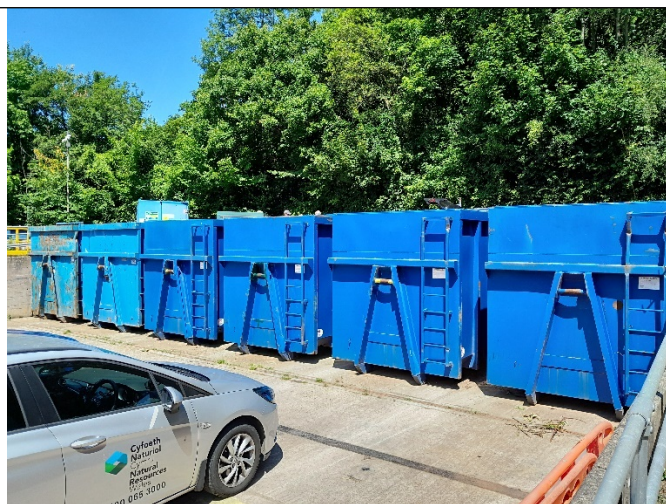
Photo 3 – Infrastructure in good condition
