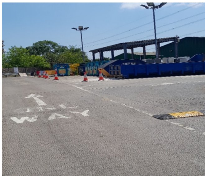
Photo 1 – HWRC area – good infrastructure
