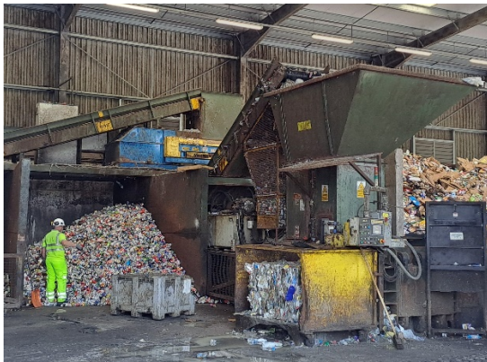
Image 3 shows MRF machine used in line with permit conditions and staff wearing appropriate PPE for transfer station working.
