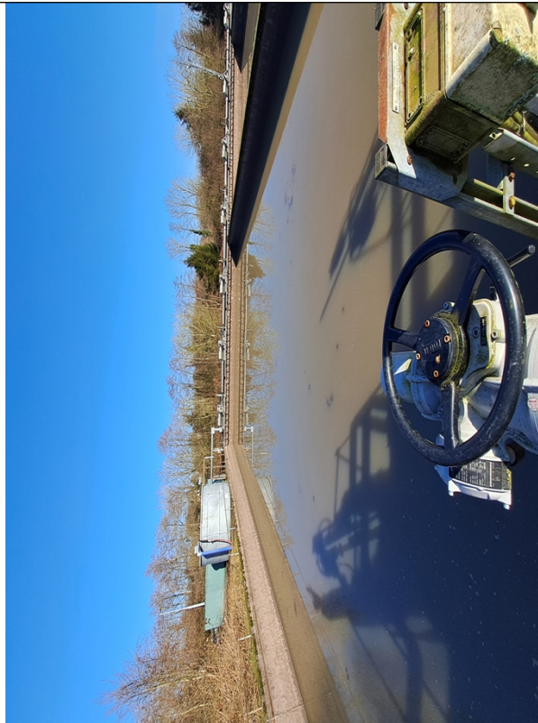
Figure 13 – Storm Tank 1 as observed during the visit.
