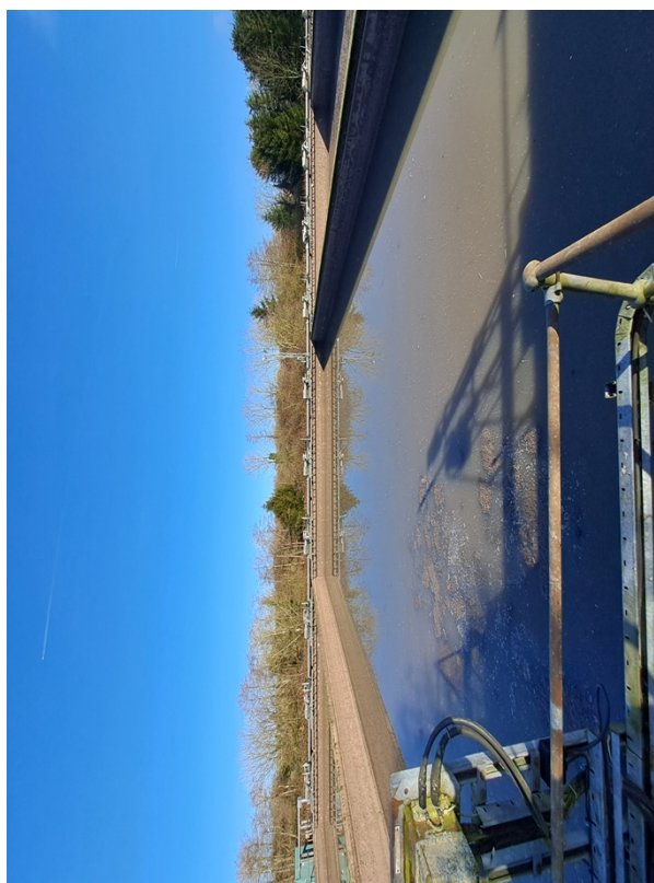
Figure 15 – Storm Tank 2 as observed during the visit.
