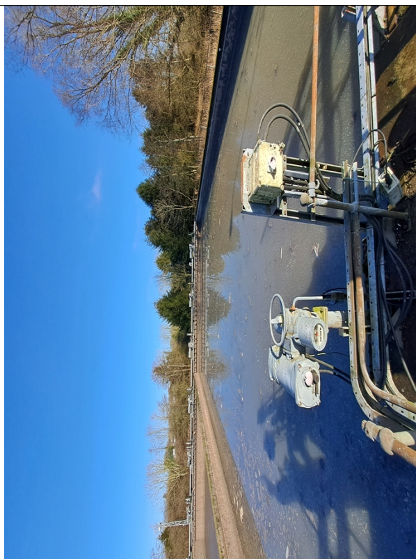
Figure 19 – Storm Tank 4 as observed during the visit.
