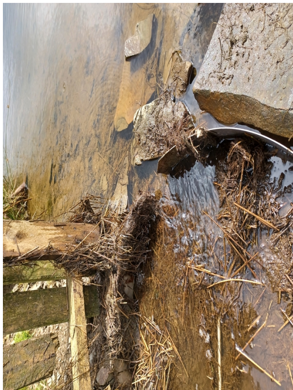
Image 3: Flow restored through notch after removal of wood and large stones.
