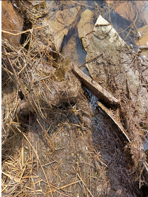
Image 2: Piece of wood and large stones arranged around and blocking Hands off flow notch
