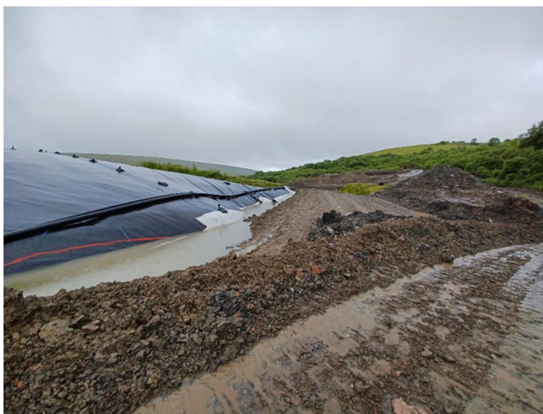
Image 1: Tie-in location at base of former access road
