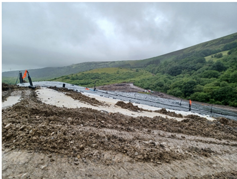
Image 3: View from crest of Tip 890 - facing Southwest
