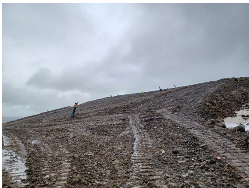
Image 2: 1000mm restoration soils deployed on the Western flank of Tip 890.
