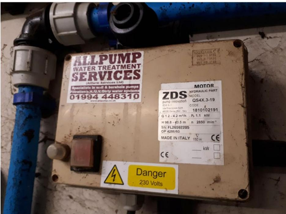
The pump installed at Point B is a ZDS X.3-19.H3F.1.5 and has a maximum capacity of 4.2m<sup>3</sup>/hour.
