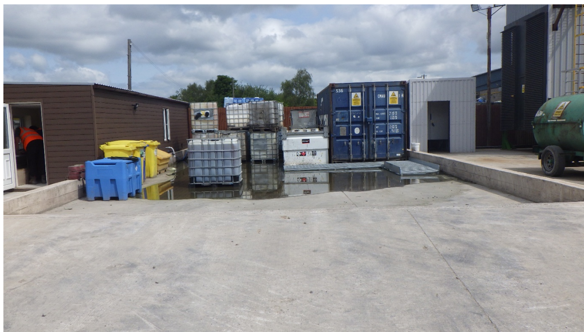
Photograph above of Fuel storage area.
