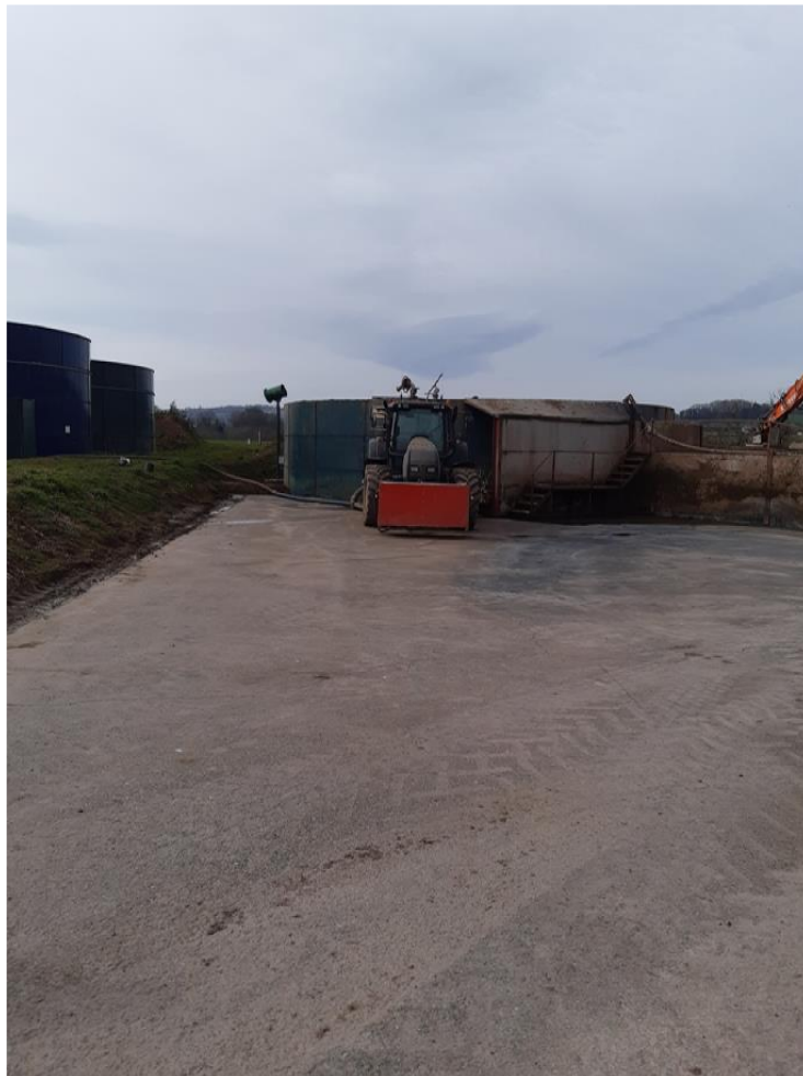
Image 1: Glass coated panelled storage tank.
