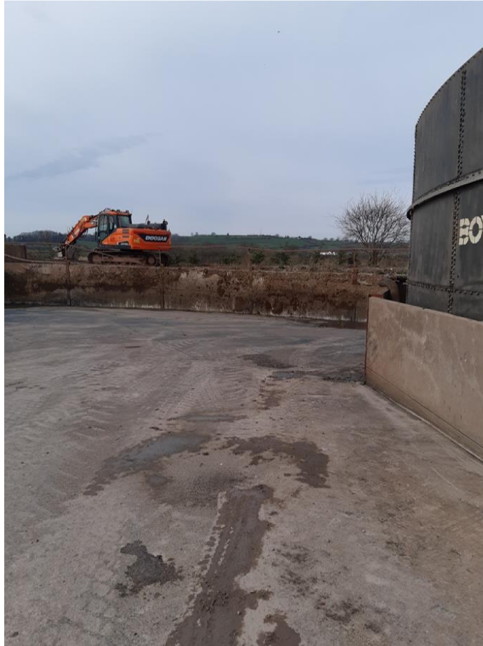
Image 2: Concrete area including Bunding
