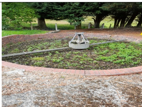
Image 2 – filter bed in need of maintenance
