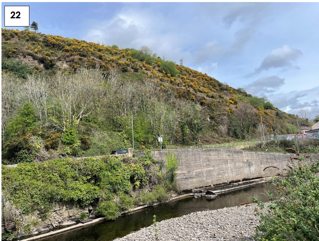
Photograph A21 & A22: River Afan to the north of the site
