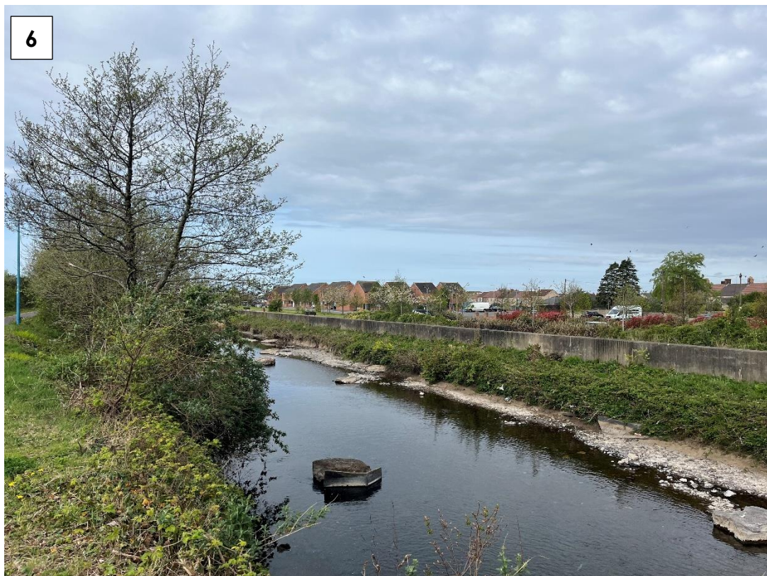
Photograph A5 & A6: River Afan
