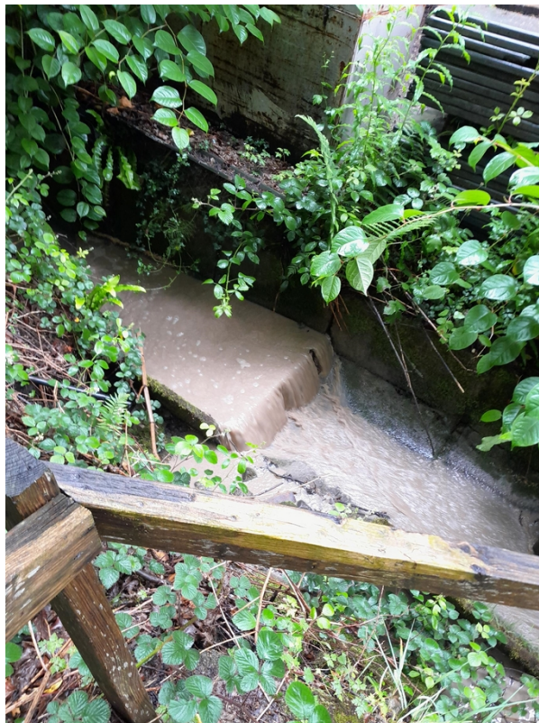
Figure 1: The discharge as it appeared during EAAT's routine sampling visit on the 05/06/2025.
