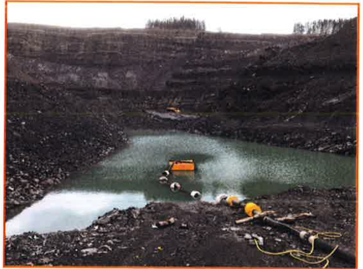
Main Void sump with submersible pump
