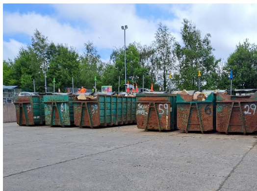
Image 2 shows site yard and waste bays in good condition with no waste outside permitted areas.
