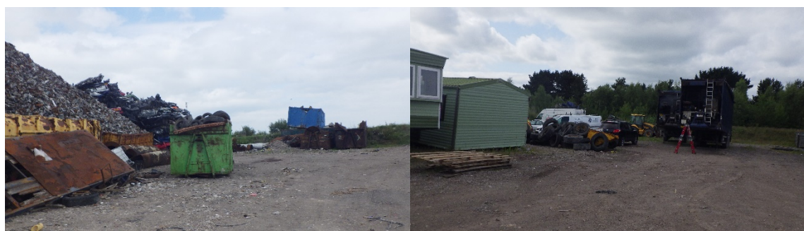
Tyres stored in a metal skip on permeable ground and in a pile on permeable ground
