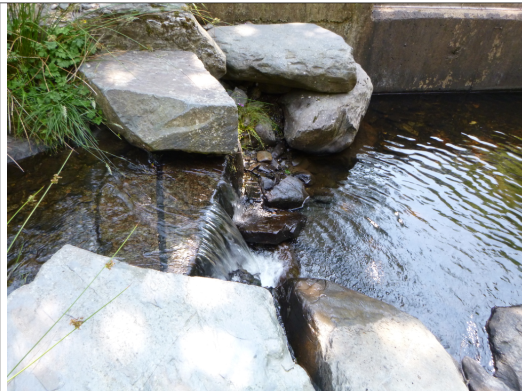
Photograph 5: Water flowing from Fish Pass into Plunge Pool (6th July 2018)
