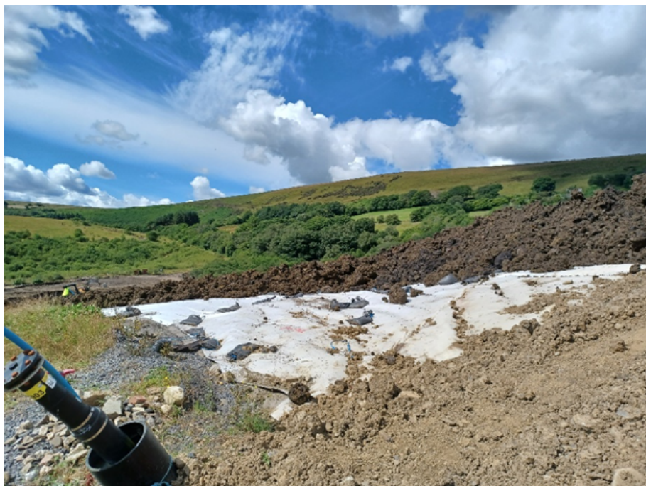
Image 2: Final section of exposed Geocomposite Drainage Layer (GDL) awaiting deployment of restoration soils
