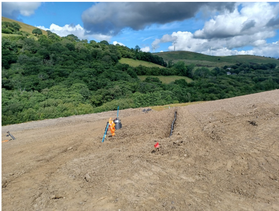
Image 4: Partially completed spinal drain associated with surface water drainage system.
