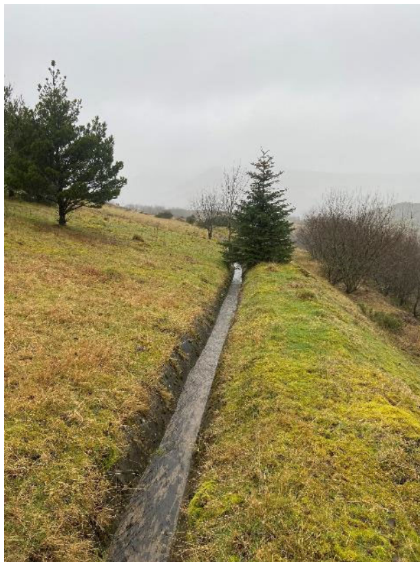
Concrete drainage channel
