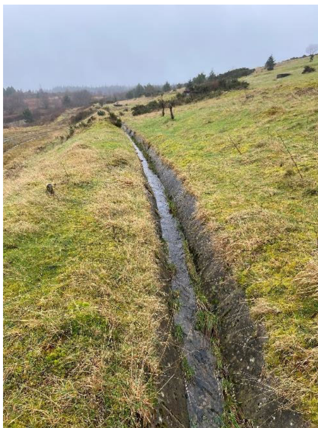
Concrete drainage channel
