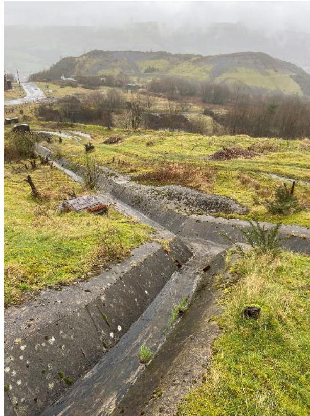
Primary drainage culvert
