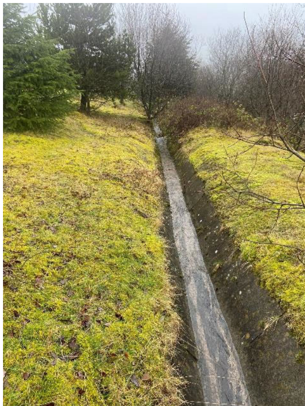
Concrete drainage channel
