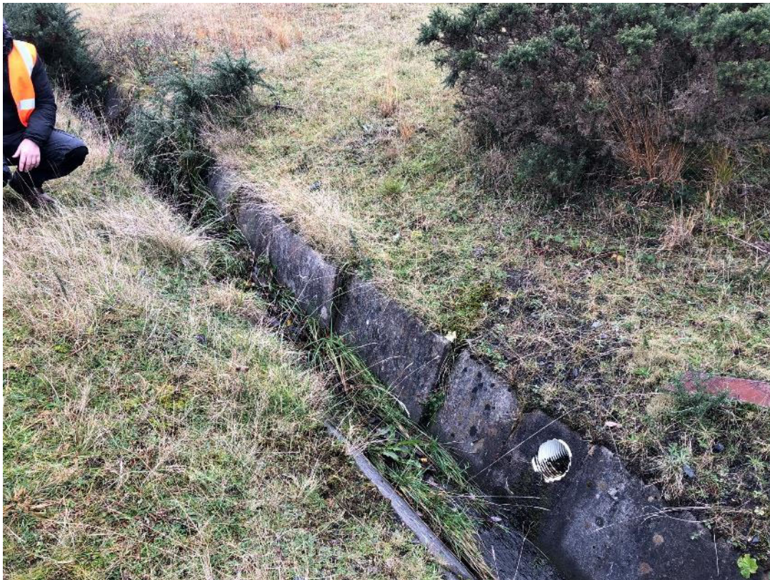
Concrete drainage channel
