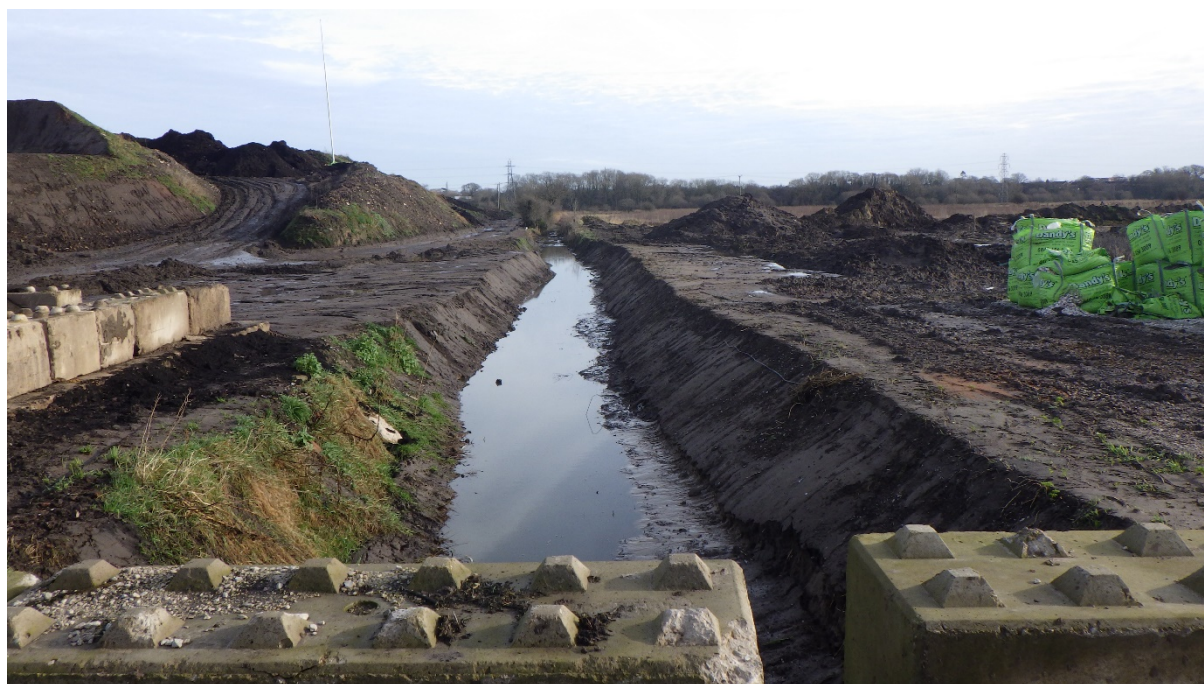
Photo from previous inspection, only for reference.
