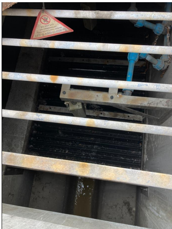
Fig 5. site visit with CSO maintenance team 21/06/2024
