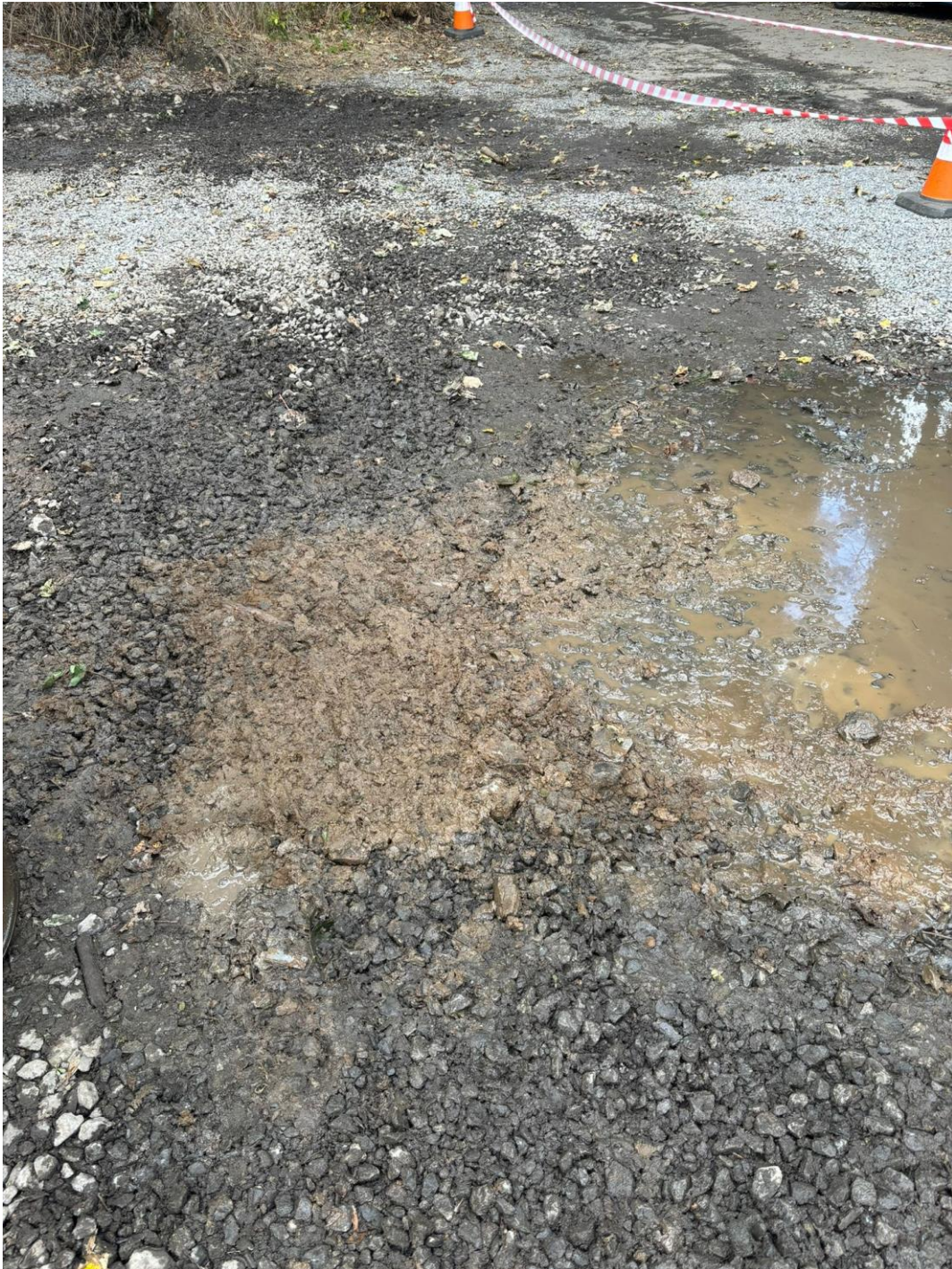
Figure 5 - Test pit remediation
