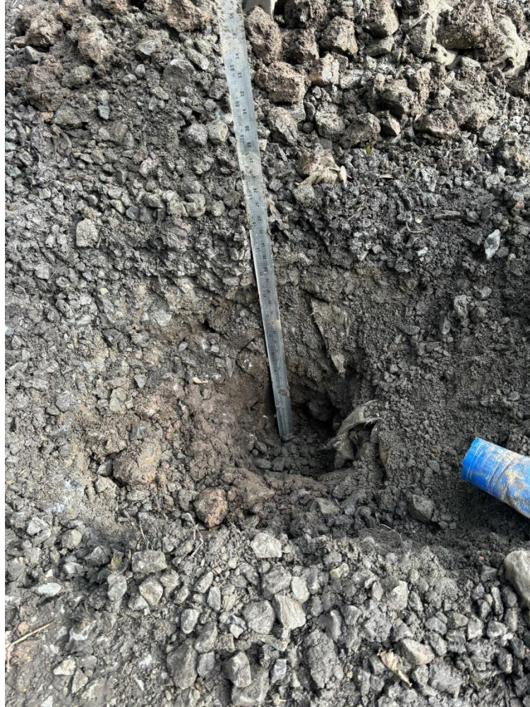
Figure 2 - Test pit F1 during excavation
