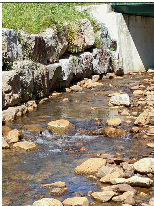
Photograph 3: Upstream View of Weir Locations 4&5 (Points D&E)
