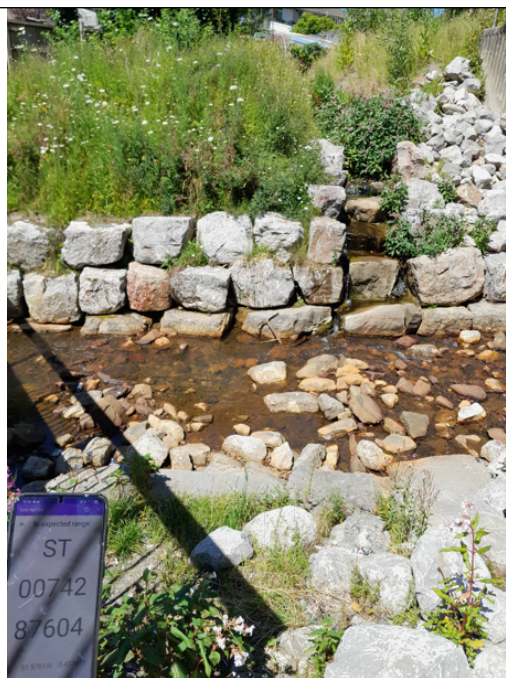
Photograph 1: Point B Block Stone, Riprap and Cascade
