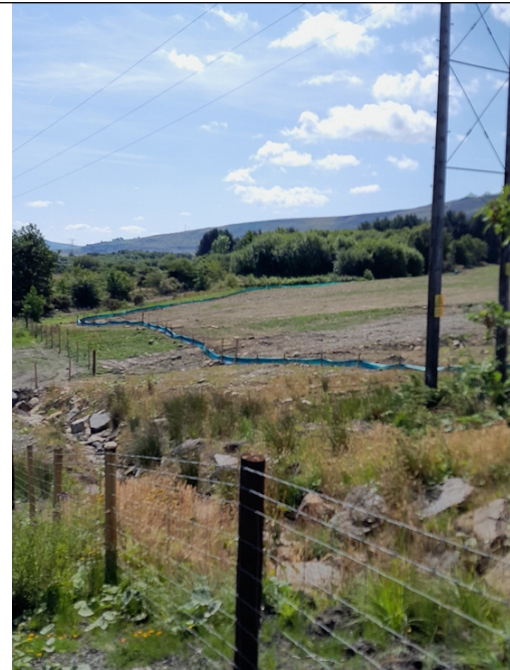
Photograph 2: Silt Fencing Being Installed
