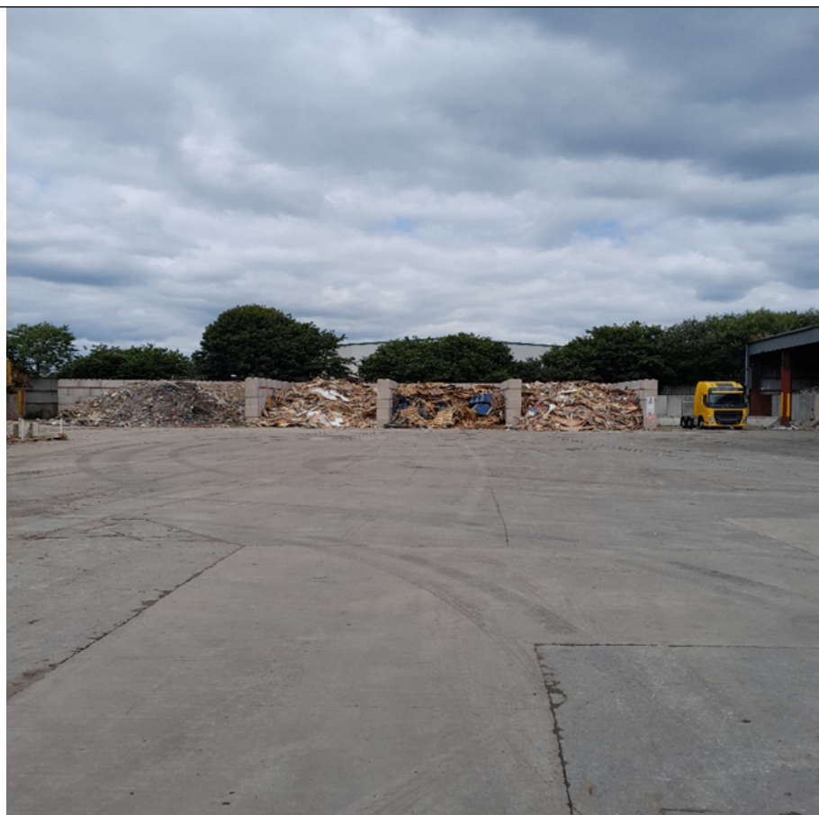
Photo 1 – New bays constructed containing wood and trade waste.
