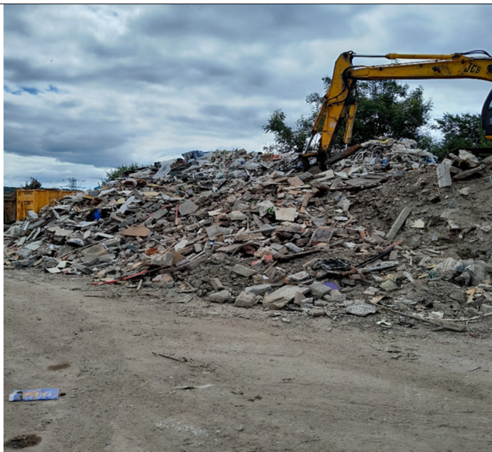
Photo 3 - Stockpile of general waste being processed.
