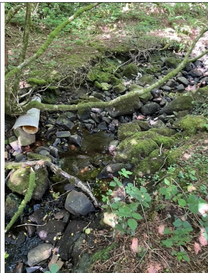
Figure 4: Nant yr Hafod downstream of abstraction and intake infrastructure
