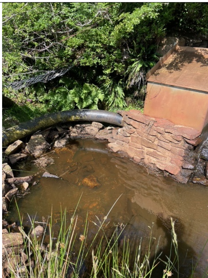
Figure 2: Intake Works- Gravity feed penstock pipe
