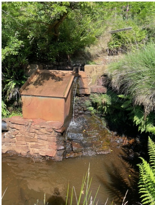
Figure 1: Intake Works- Concrete Weir
