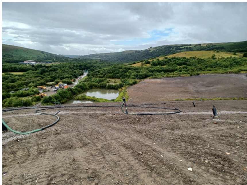
Image 2: View from crest of Tip 890 – facing south. Area previously awaiting restoration soils now completed.
