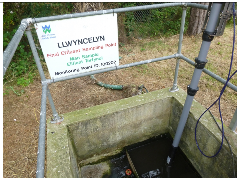
Photograph 2: Final effluent sampling point
