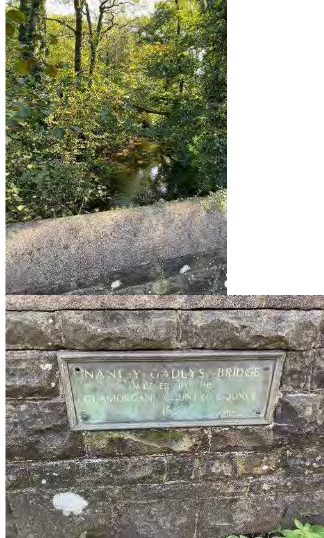
A4063 bridge running over Nat y Gaeltach
