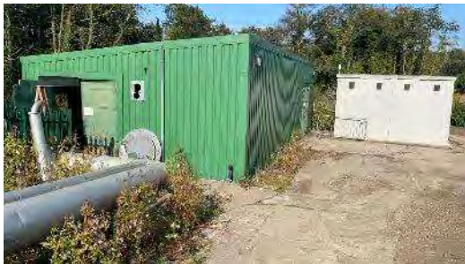
Abstraction Point A – not signed but presume building is abstracting water.
