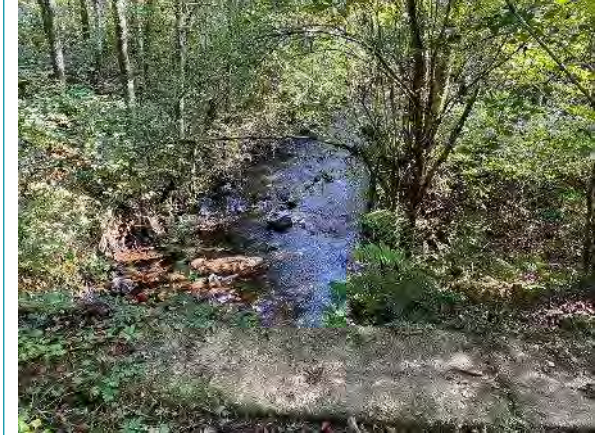
Foot bridge over Nat y Gaeltach
