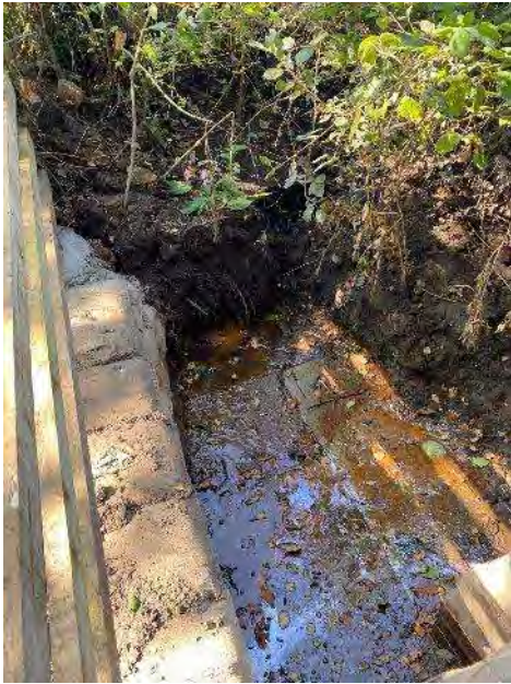
Man made water drainage underneath B road. Very little water
