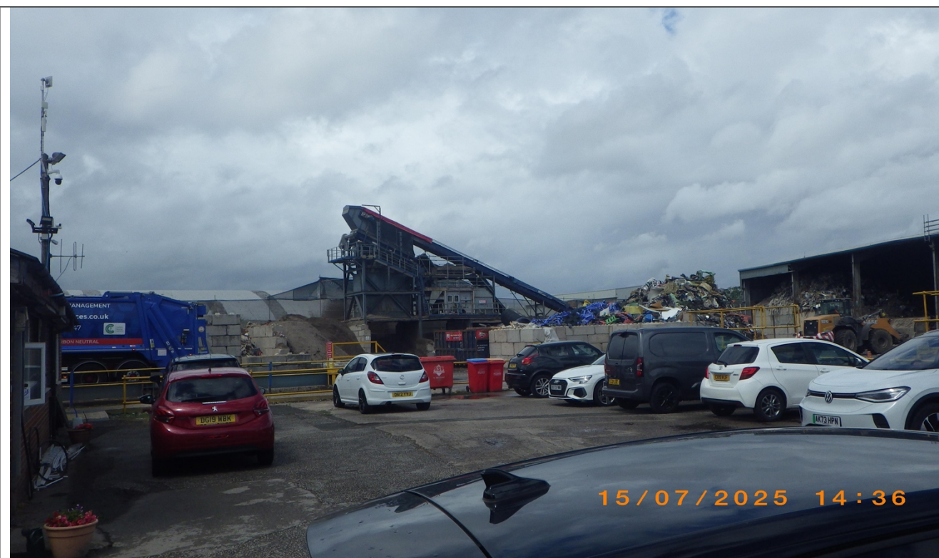
BlueMAC machine with centre conveyor belt cover missing.
