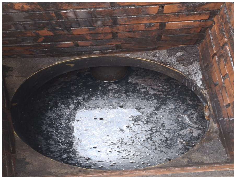
Figure 3: Interior of final interceptor chamber before discharge
