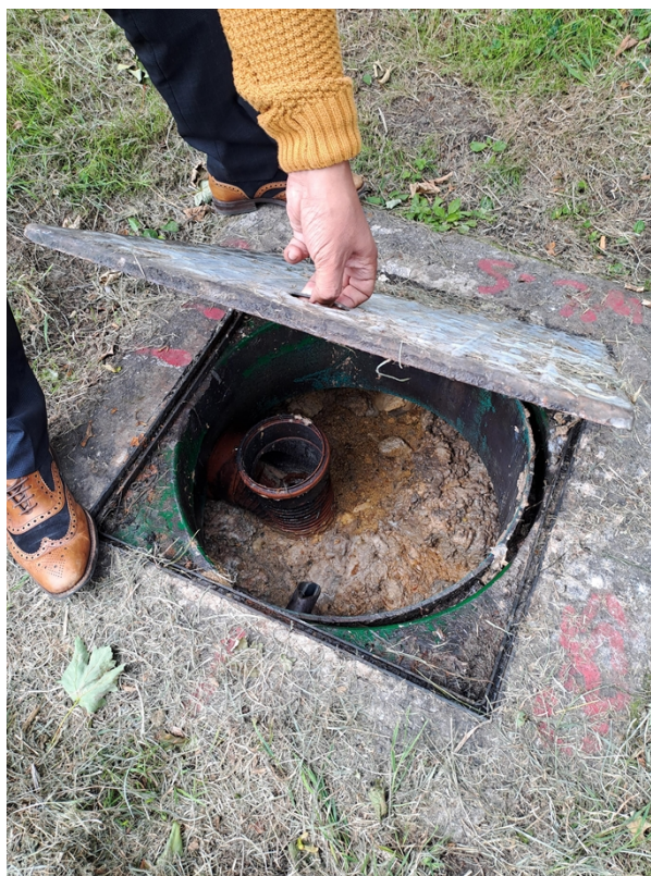
Figure 1 – Chamber 1 of the treatment plant as observed during the visit.
