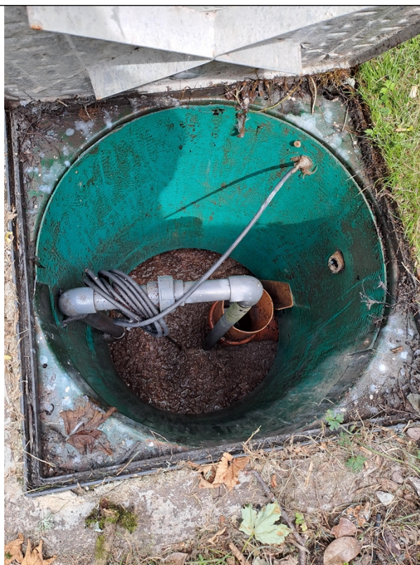
Figure 4 – Chamber 4 of the treatment plant as observed during the visit.
