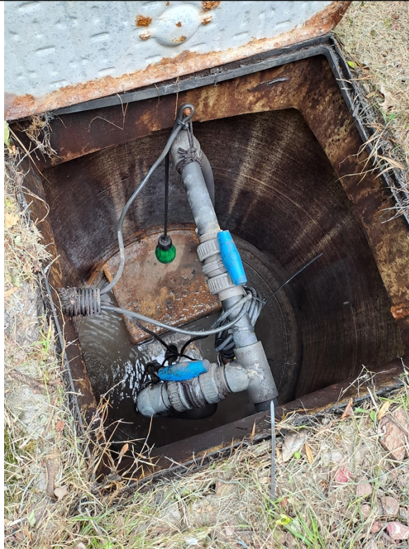
Figure 5 - Chamber 5 of the treatment plant as observed during the visit.
