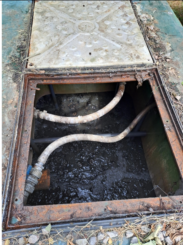
Figure 3 – Chamber 3 of the treatment plant as observed during the visit.
