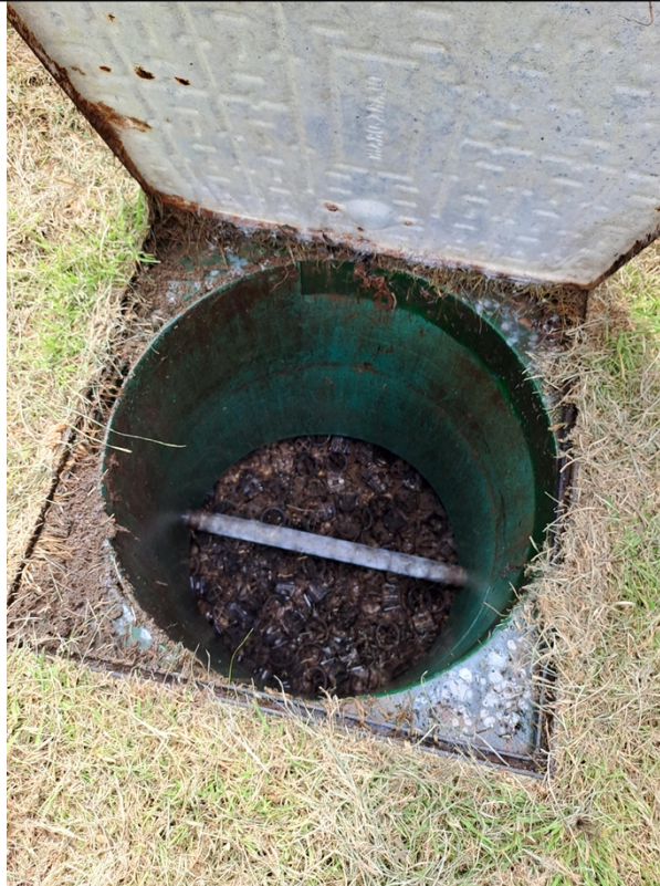
Figure 2 – Chamber 2 of the treatment plant as observed during the visit.
